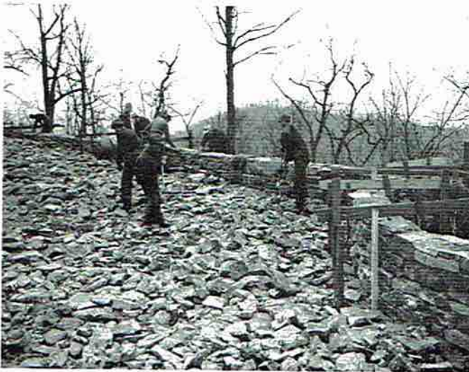
Construction of parking area.
