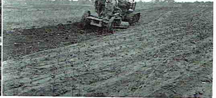
Tractor and grader in operation.
