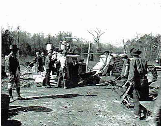
Construction on a 100-acre lake.
